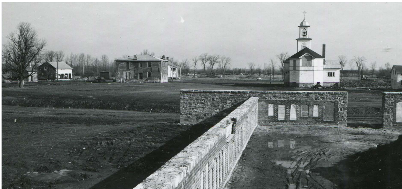
The Pioneer Memorial and parts of Upper Canada Village during its construction in 1957. The best tombstones from the Lost Villages were selected and carefully encased in brick walls, preserving them for future generations. (Lost Villages Historical Society)
